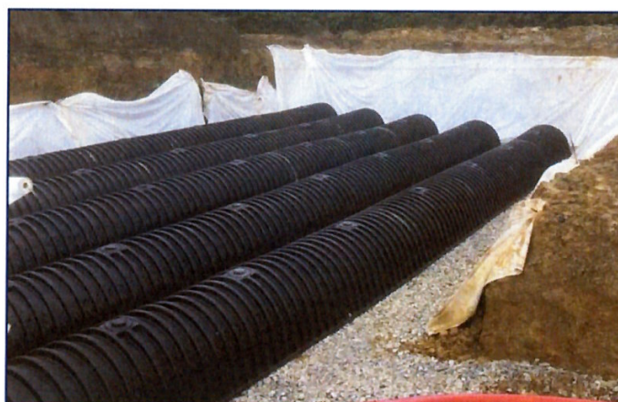
Figure 3.8 – Typical Poly-Tunnel Installation Arrangement
